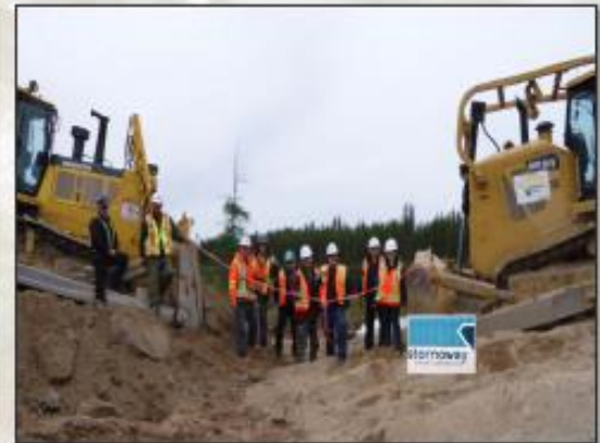
Connection of the Renard Mine Road September 2013
