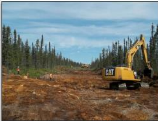
“Slashing” or Tree Clearing
