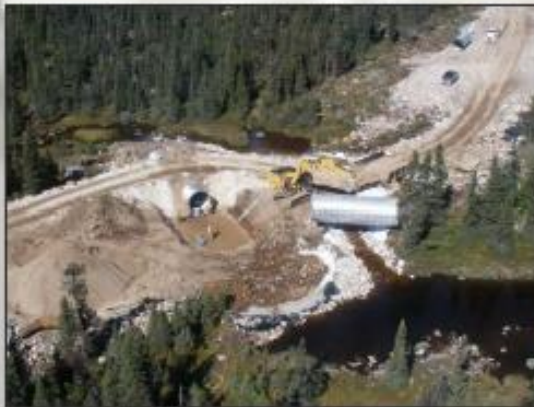
Bridges or Culverts on Stream Crossings
