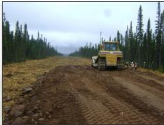
Preparation of Road Foundation
