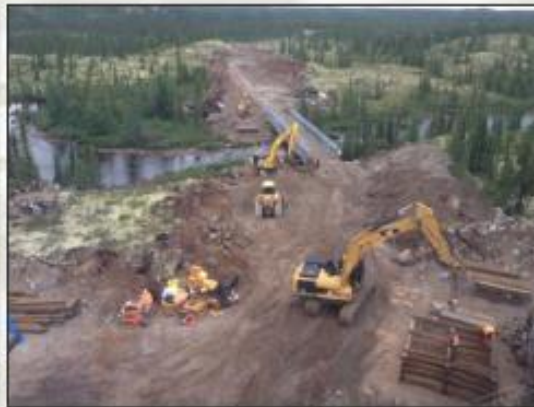
Construction of Permanent Bridges
