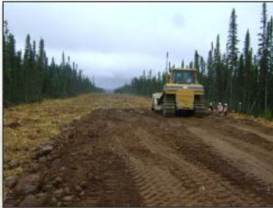
Preparation of Road Foundation
